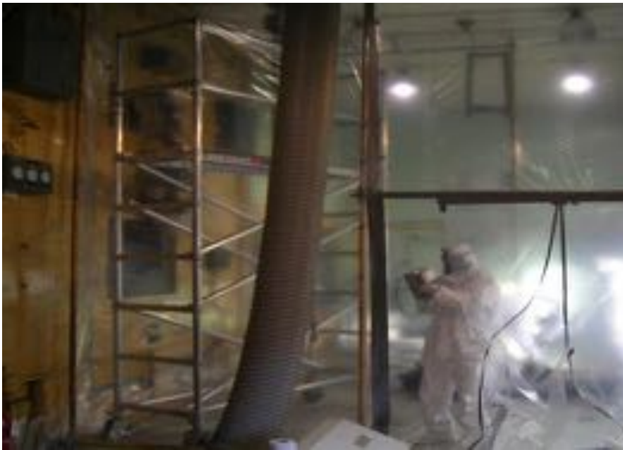
Working area isolation and Air monitoring
