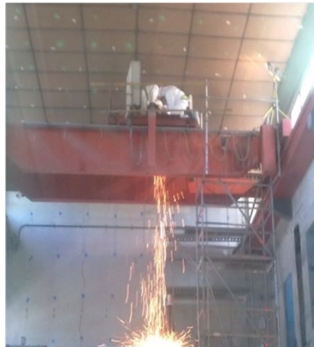
Crane dismantling
