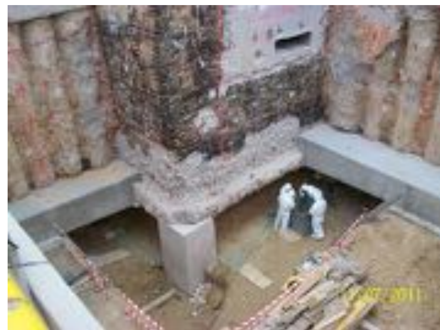
Excavation reached 10 m deep
