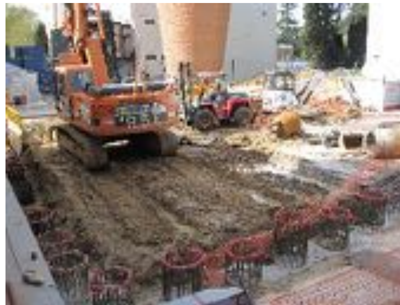
Pile foundation for safe excavation
