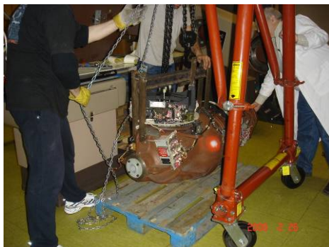
Figure 2 Removal of the head of a teletherapy equipment with Co-60 source.
