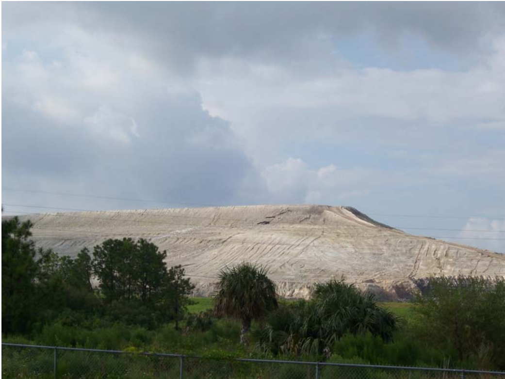
Figure 2. Phosphogypsum stacked on land.
