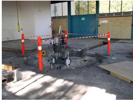
Figure 27. The measurement at the reactor foundation area.
