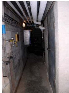
Figure 7. One of the rooms in the eastern basement.
