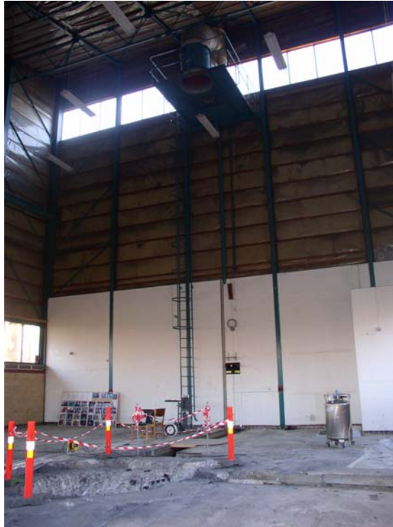
Figure 23. Measurement on the ventilator channel.
