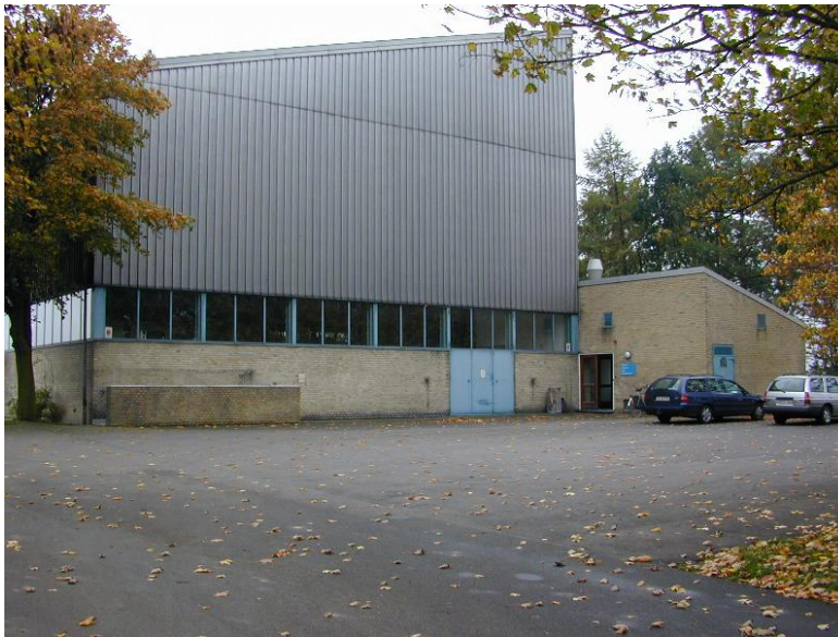
Figure 9. The DR 1 building seen from north-east. The asphalt in front of the building is classified as a class 1 area, staircases leading to the basements are classified as class 2 areas, while the rest of the land areas in the vicinity of the reactor building are regarded as non-classified.
