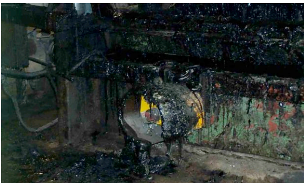
Figure 6: Challenging environment, but in this case the gauge is protected by a mudguard and a trefoil warning sign was placed to the right of the picture.
