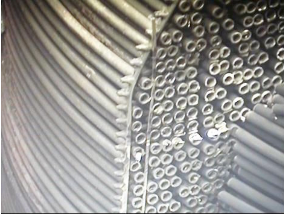
Fig. 3 Tube bundle cut into pieces.
