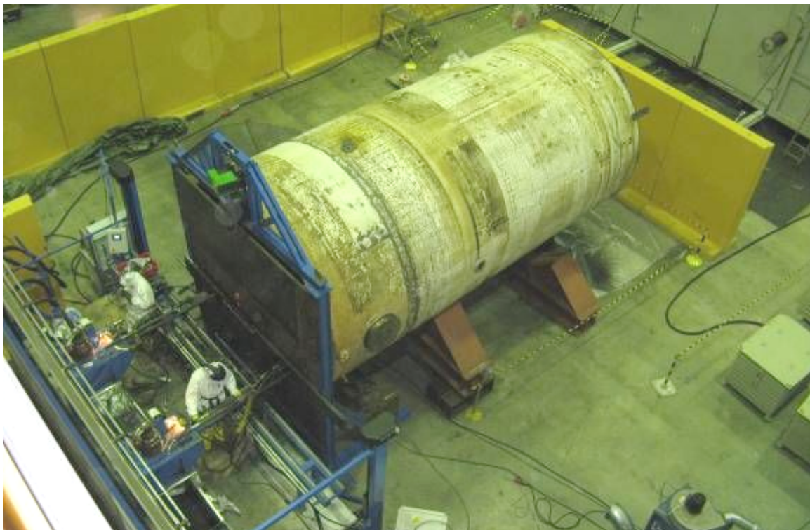
Fig. 3 View tube pulling
