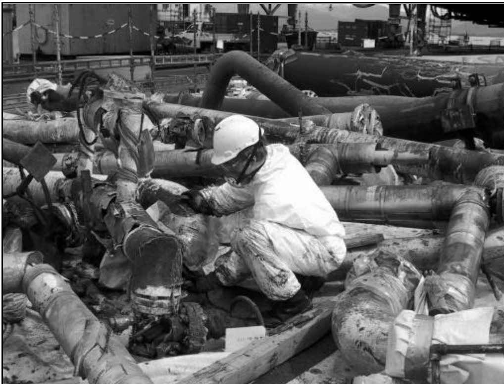
Figure 2. Identification of LSA Scale contaminated tubes during decommissioning of an oil producing platform.
