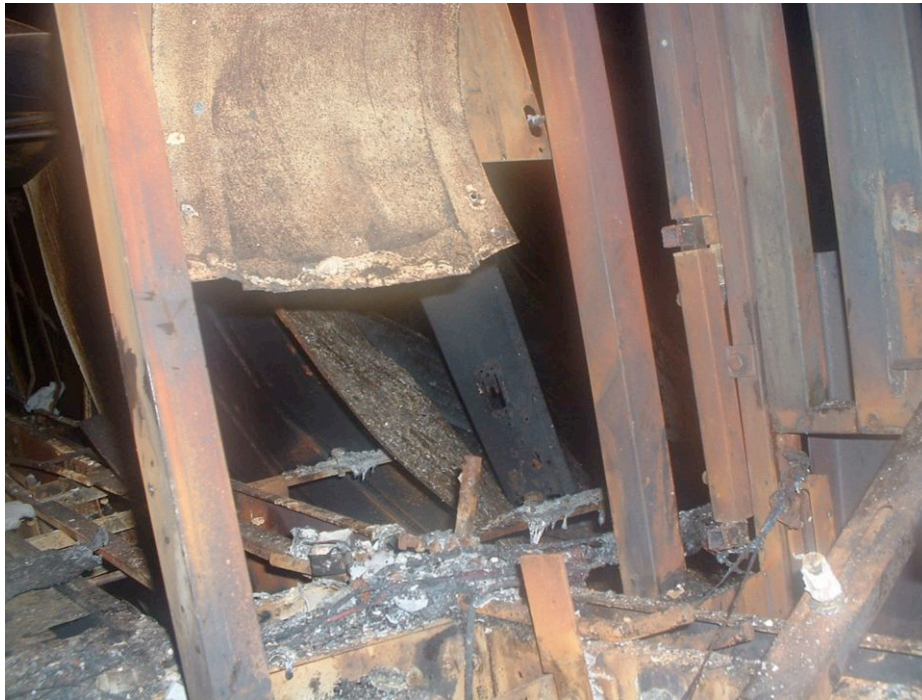
Figure 2. Portion of galvanised sidewall that was cut through by fire crew to facilitate access to the production line area
