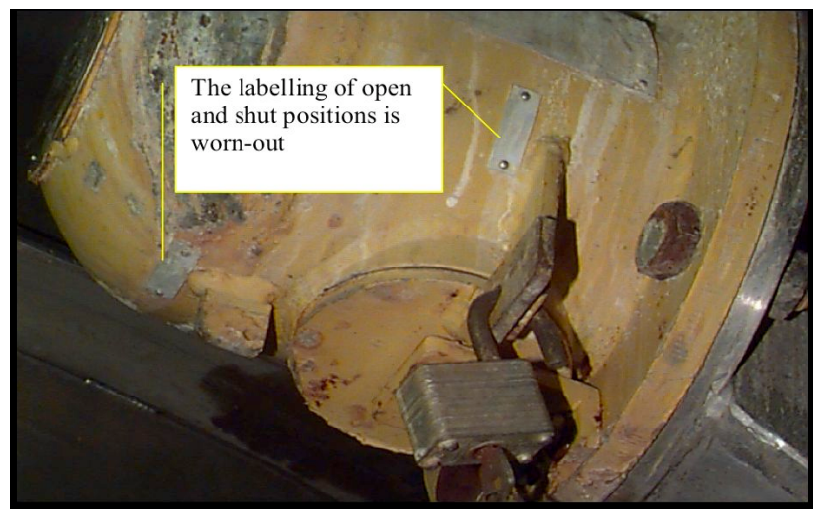
Figure 5: The labelling of open and shut position is worn-out.
